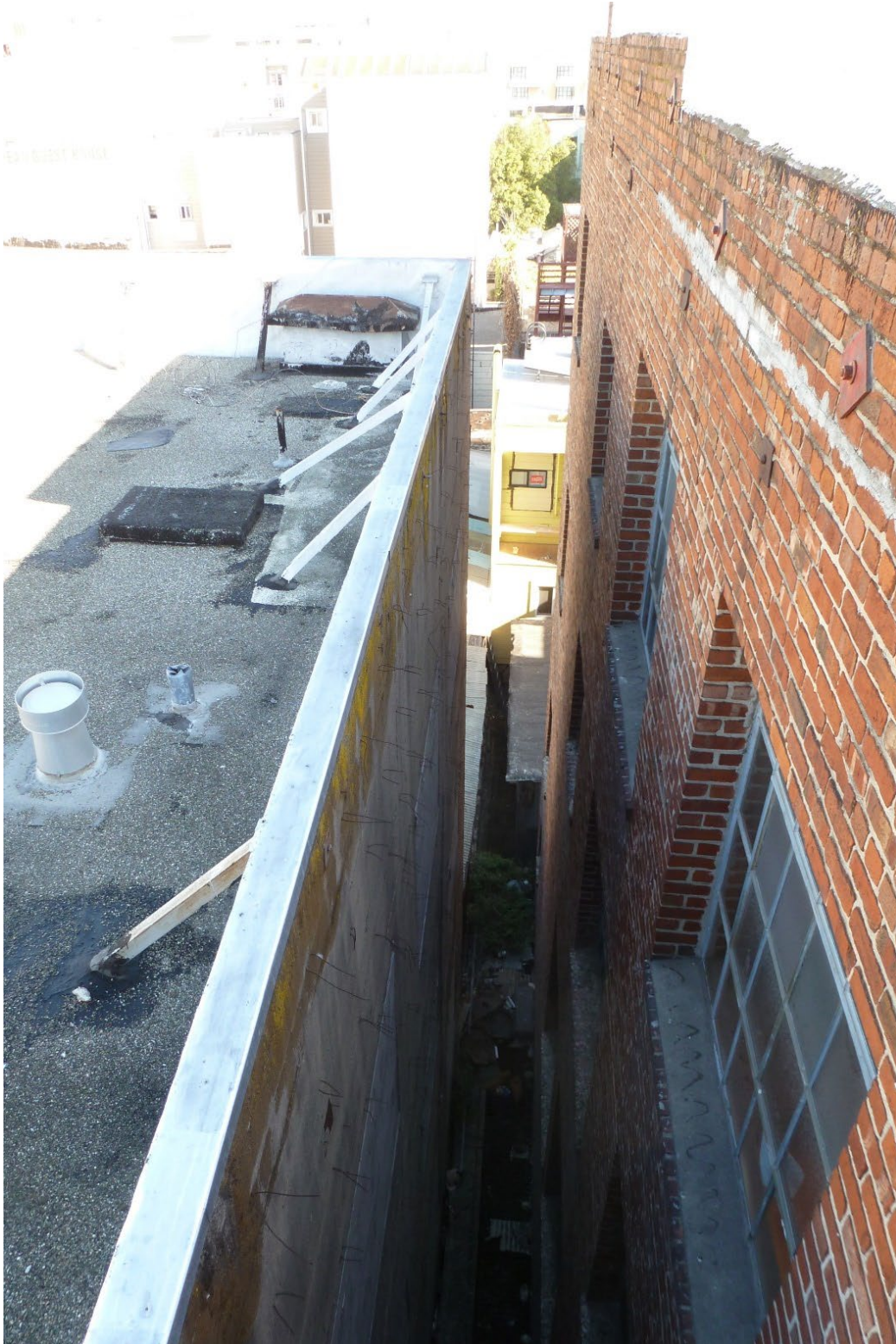
Photo 11 View of northwest façade from rooftop. Looking northeast.
