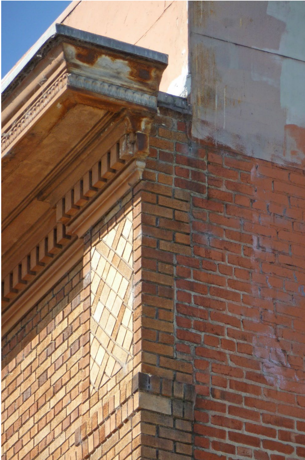
Photo 12 Detail view of cornice at the east corner. Looking west.
